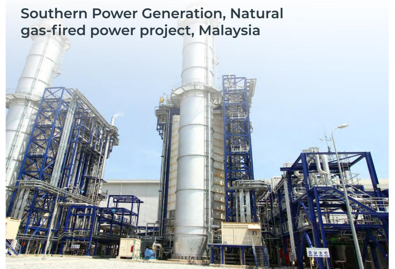
Developed by Southern Power Generation (SPG), this 1.44GW plant is equipped with advanced power technologies, including the world's first GE 9HA.02 gas turbines, specified for their high efficiency and low carbon emissions.
